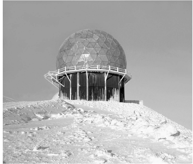
FIGURE C. A 55-ft-diameter rigid-space-frame radome installed atop an arctic tower at Thule, Greenland. Note the absence of significant radome icing.
