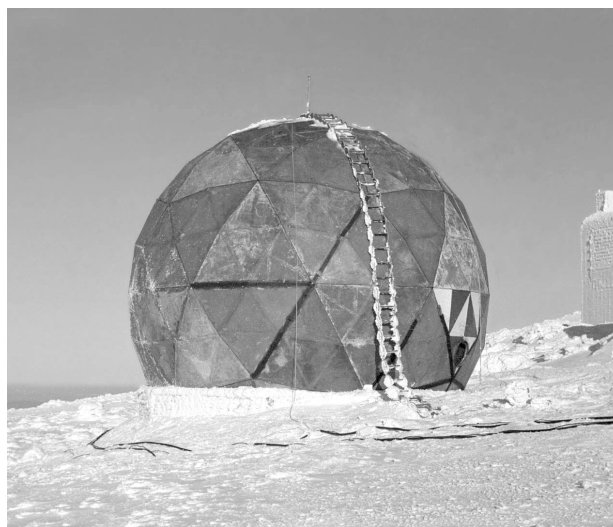
FIGURE A. Lincoln Laboratory's first 31-ft-diameter rigid-space-frame radome, used near the summit of Mount Washington, New Hampshire, for environmental testing. Most of the surface panels are equilateral triangles. Note that there is not much rime ice on the radome, compared with the nearby building. Any accumulated ice was easily removed by internal heating and dragging ropes across the radome's exterior.
