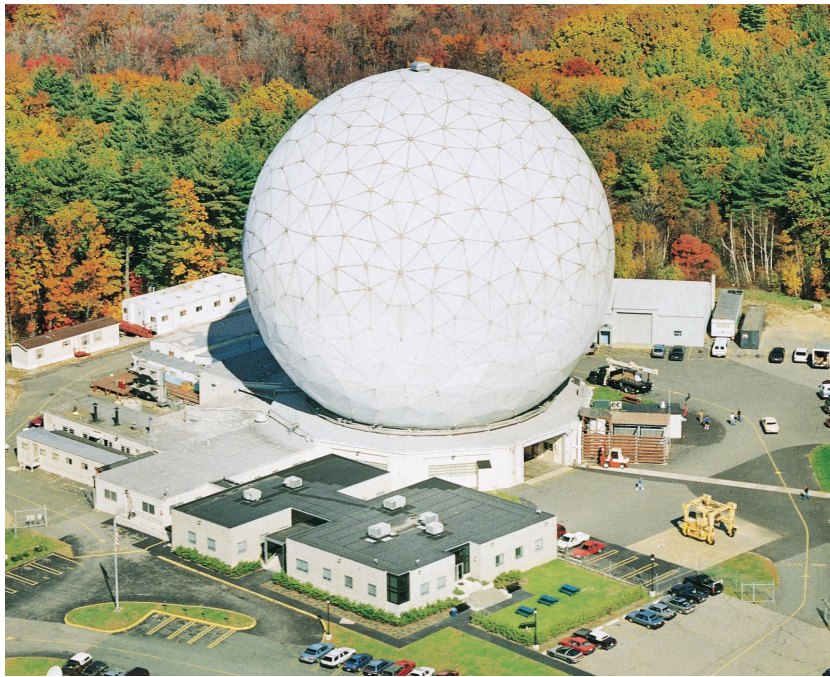
FIGURE F. The 150-ft-diameter rigid metal space-frame radome at Haystack Hill, Tyngsboro, Massachusetts.
