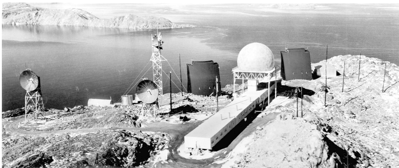
FIGURE 13. A representative DEW Line radar station at Baffin Island, Canada. The rotating antenna of the L-band AN/FPS-19 radar is housed in the 55-ft-diameter rigid-space-frame radome, which straddles the “railroad-train” array of wanigan shelters in which the station’s crew lives and works. The two fixed receiving antennas of the UHF AN/FPS-23 bistatic Flutter radars are mounted on the tall tower in the middle of the picture, each aimed toward an adjacent unmanned Flutter-radar transmitting site. At left are two circular paraboloidal antennas for communication with other stations along the line. Visible at the right are two rectangular paraboloidal reflectors of an AN/FRC-47 terminal for longer-range communication. Both communication systems rely on UHF tropospheric scatter. (Image property of AT&T Archives. Reprinted with permission of AT&T.)
